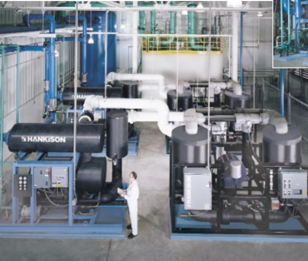
Three 9000 scfm (255m<sup>3</sup>/min) Hankison HEDS Series Drying Systems furnish clean, dry air to a major automobile assembly plant.
